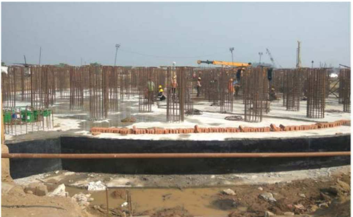
Ammonia Storage Tank-B under Construction at HURL Gorakhpur.
