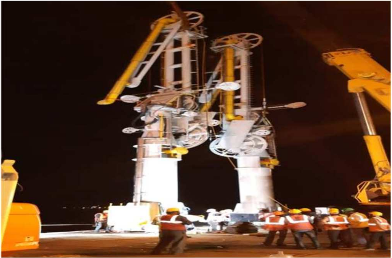
MARINE LOADING ARMS ERECTED - LPG TERMINAL MUNDRA
