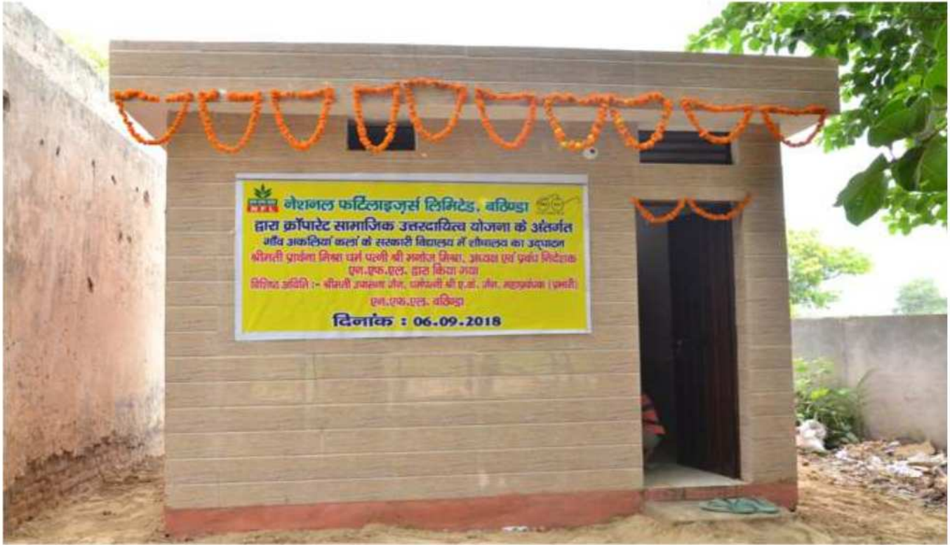
Toilets have been constructed by NFL under Swachh Bharat Abhiyan as CSR activity at Govt. Schools in villages near Bathinda Unit.
